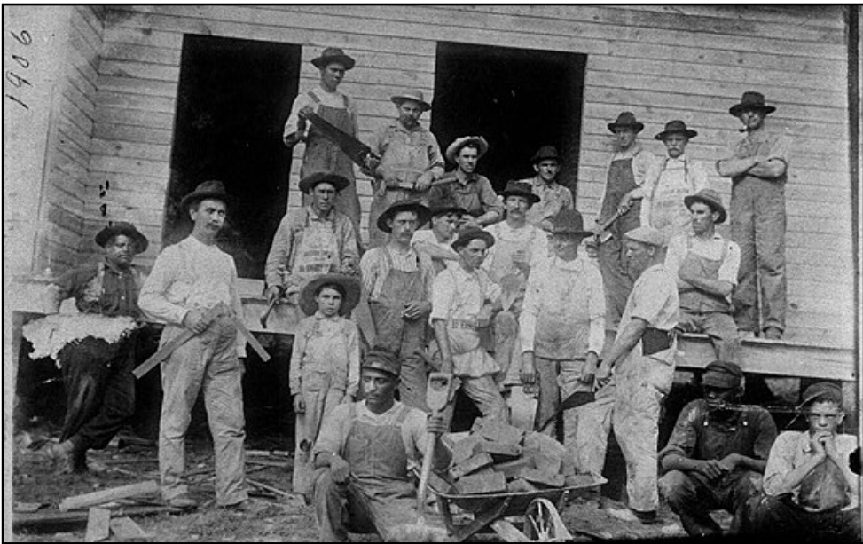
Plainville house construction, ca. 1900: Workers in the process of constructing a house pause to pose for a photograph. Note the tools and the wheelbarrow filled with bricks. (Vanishing Georgia, Georgia Archives, Morrow, Georgia.)
