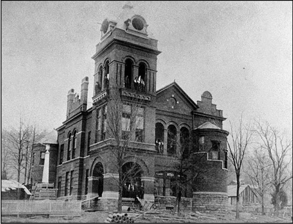
Calhoun, 1889. Gordon County Courthouse under construction. Two men associated with the building of the courthouse were William Dowling and W.L. Hillhouse. The courthouse was demolished in 1961. (Photo: VANISHING GEORGIA)
